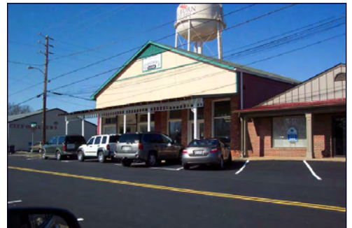
Shopfront buildings, such as the Country Store, line the northern edge of 4th Avenue.
