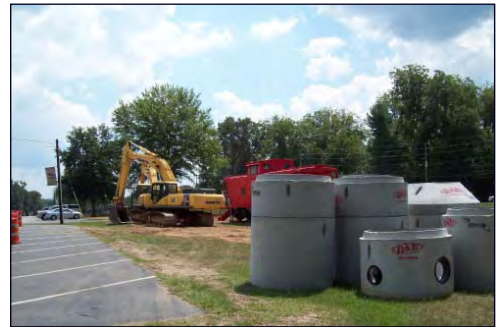
New sewer improvements installed along 4th Avenue will help accommodate new development in the downtown district in future years.
