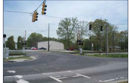
Signalized intersection at the corner of Atlanta Highway and 6th Street.
