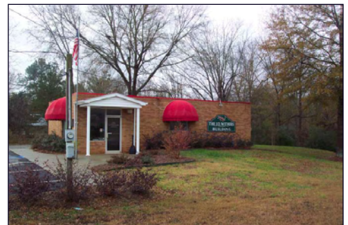
The J.D. Withers Building, located along Atlanta Highway, serves as a community center for small local events and gatherings.
