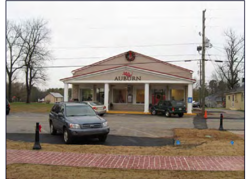
Auburn City Hall, in a contributing historic building, was rehabilitated with new additions and a roof covering.
