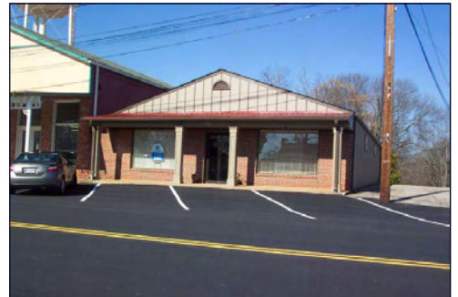
A mix of parallel, perpendicular, and parallel parking spaces along 4th Avenue provide sufficient parking for downtown civic uses and businesses.
