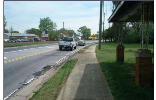
Concrete sidewalk along the south side of Atlanta Highway is separated by a small planting strip. This helps pedestrians feel safe from fast moving vehicles when walking along roadways.
